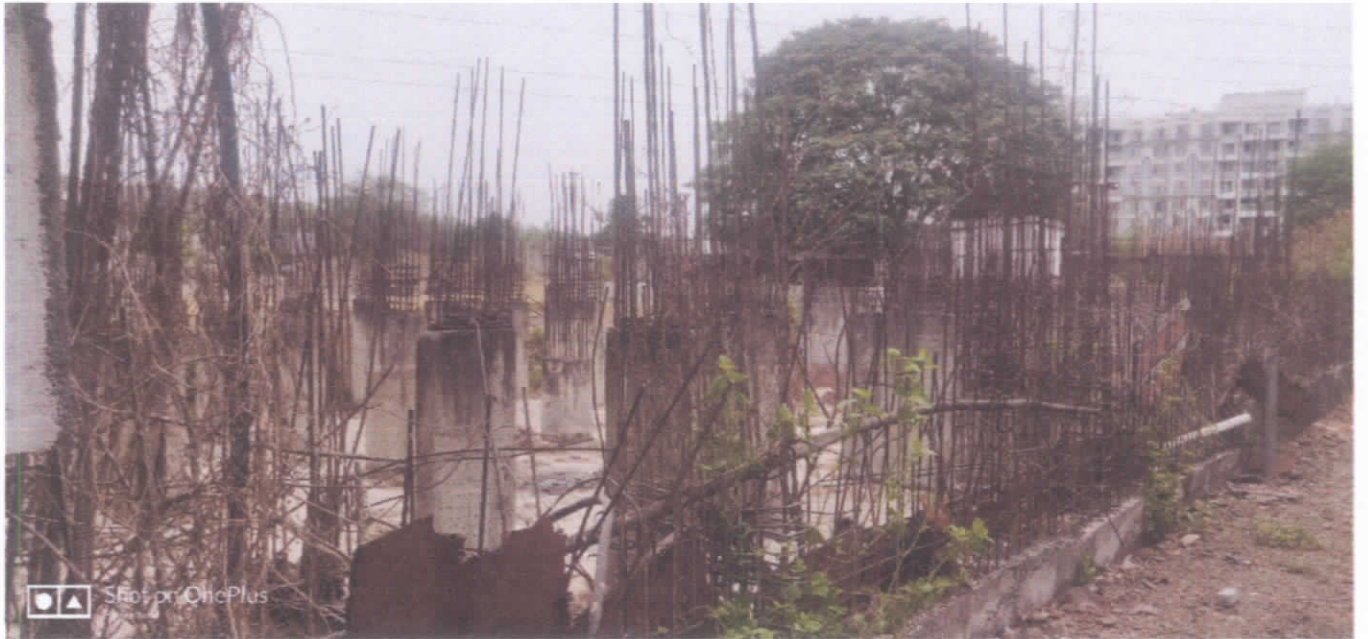
M/s Jubilee Park – Building A – Foundation and Column constructed
