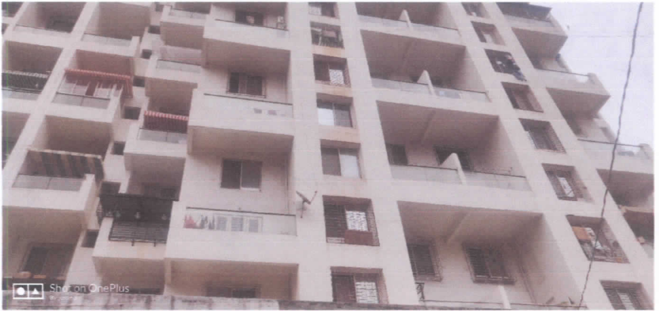
M/s Jubilee Park – Building B & C completed
