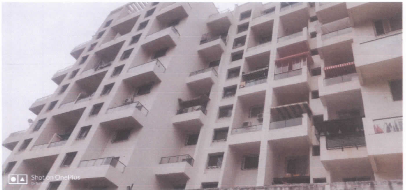
M/s Jubilee Park – Building B & C completed
