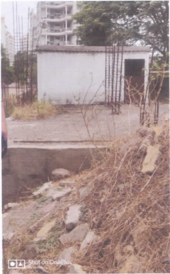
M/s Jubilee Park – Water storage tank
